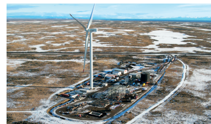
Methanol reactor for an e-fuels pilot plant being built near Punta Arenas, Chile
