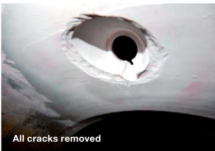
All cracks removed
