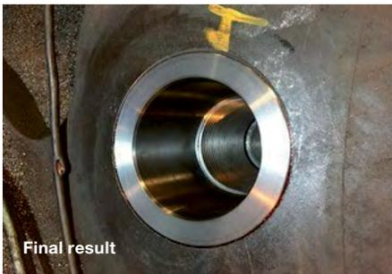
If corrosion or other unforeseen circumstances have led to a broken cylinder cover bolt or stay bolt and maybe even damages to the thread, it can be difficult or even impossible to remove the bolt. MAN PrimeServ On-site Recovery are specialists in drilling out the damaged material and restoring the tapped bore to original dimensions allowing the use of standard studs after repair.
