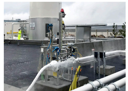
MAN W50 installed
