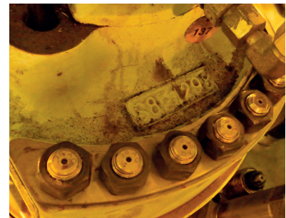
Multi-studs manually tightened from S60 and down
