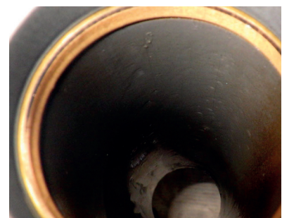
Clean and perfect spindle guide condition
