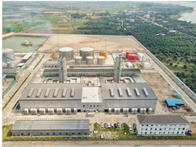
MAN Energy Solutions has commissioned a 200 MW power plant near Cambodian capital, Phnom Penh (picture source: Electricité du Cambodge)
