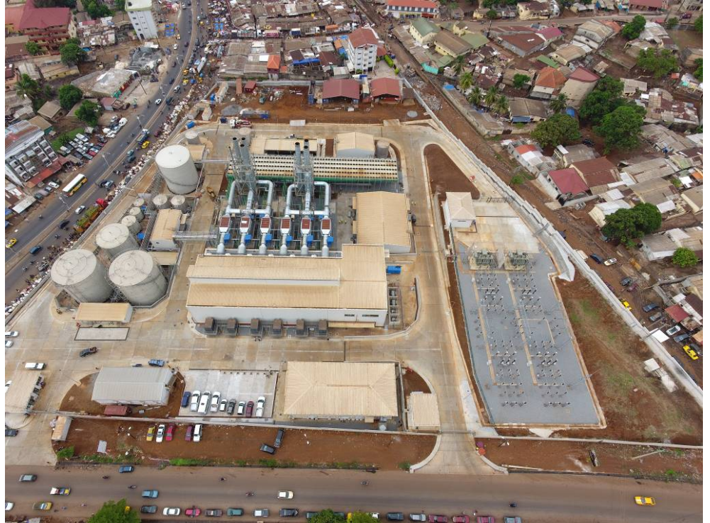
In Conakry, Guinea, MAN Energy Solutions installed 6 x MAN 18V32/40 engines in a power plant that will provide 53 MW of electrical power to the city.
