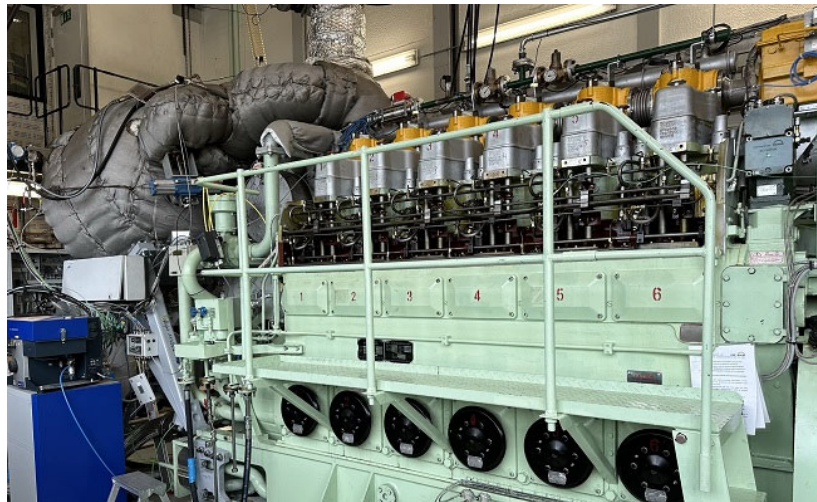
View from the testbed in Frederikshavn
