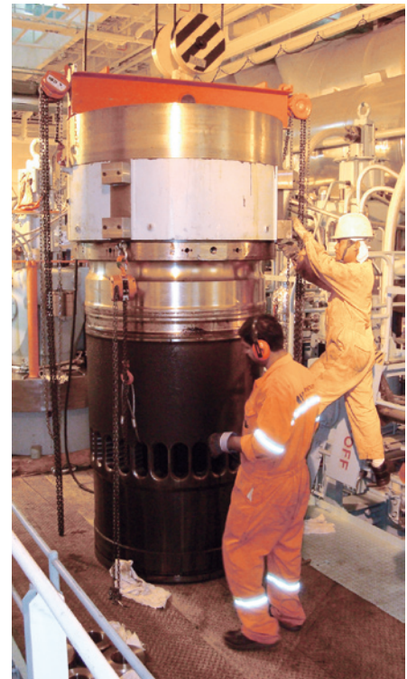
Overhaul of cylinder unit on large bore engine
